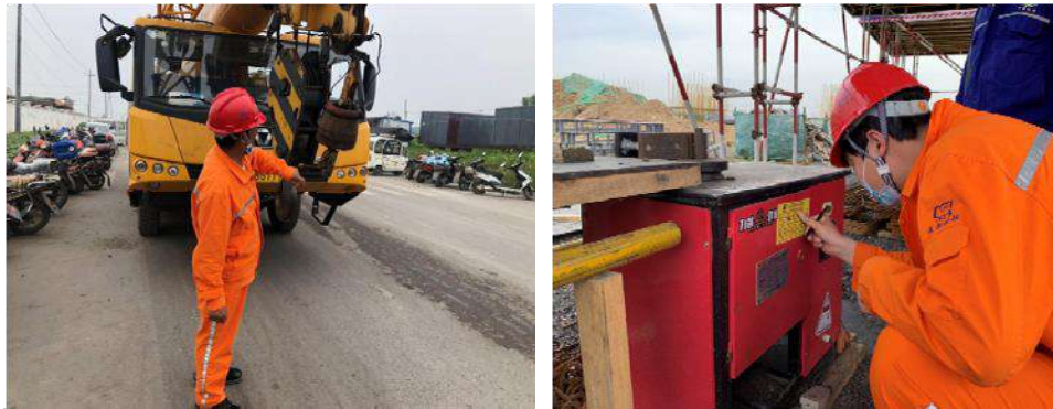
Equipment inspection and acceptance
