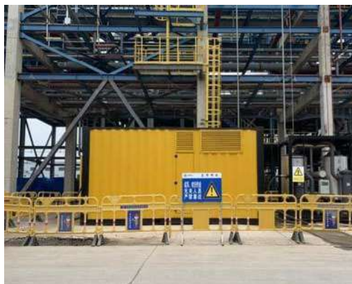
Barricade the pressure test area
