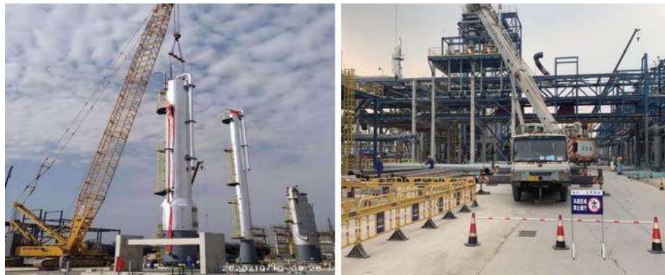
The hoisting work
