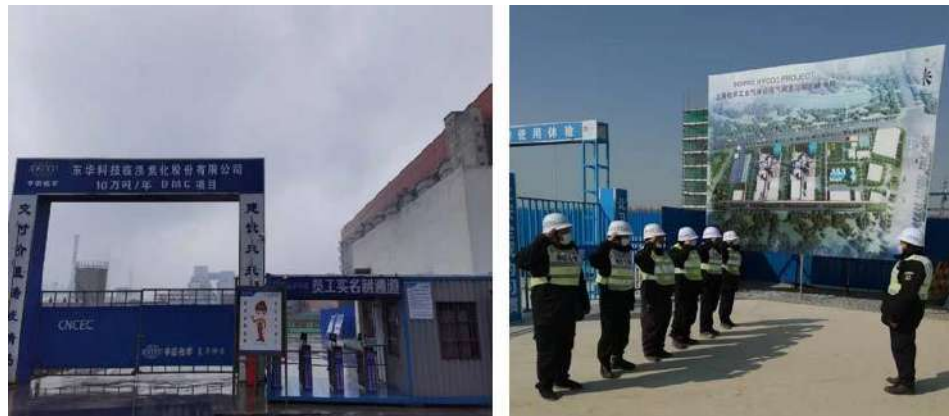
On-site access control
