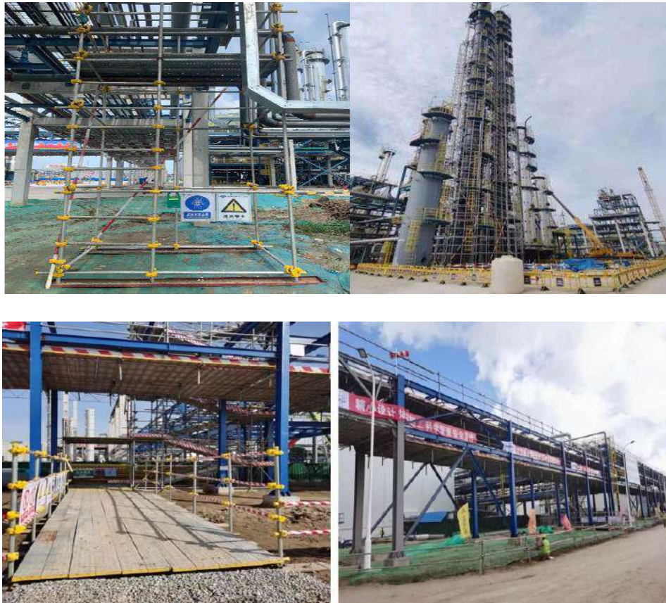
Safety protection facilities of pipe gallery construction
