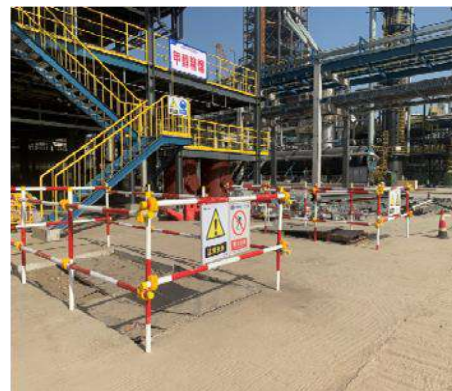
Protective barricade for foundation pit edge and holes
