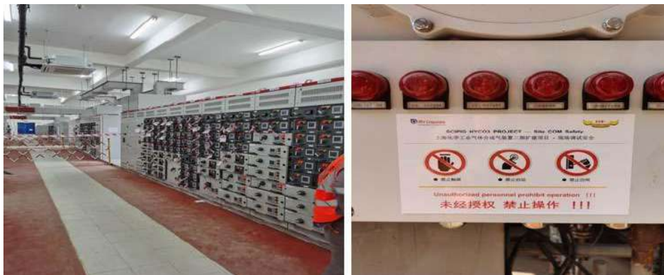
Tag-out and lock-out of electrical system commissioning
