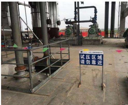
Barricade the pressure test area
