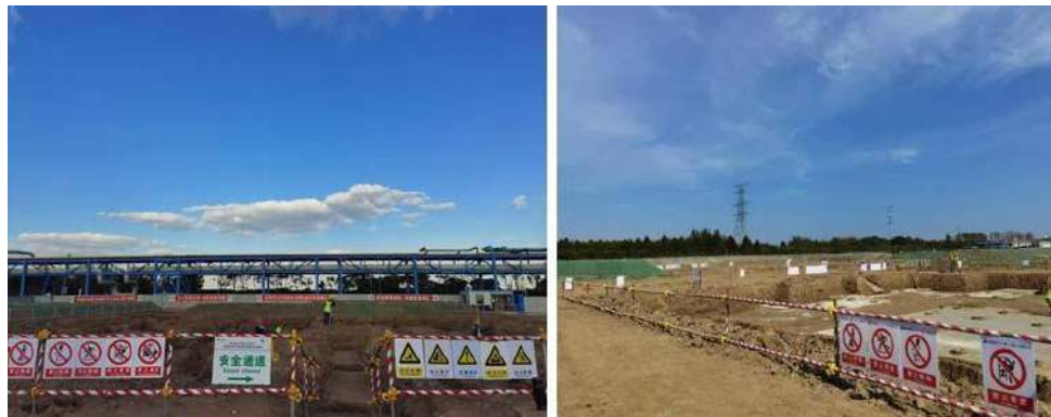
Foundation pit protection
