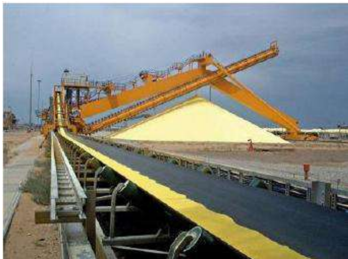
FIGURE 1.6 TYPICAL PHOTO FOR SULPHUR HANDLING AND STORAGE
