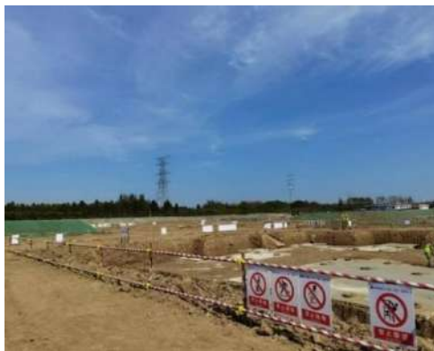
Protective barricade for foundation pit edge and holes
